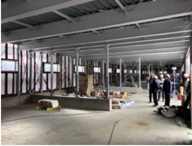
Building safety assessment
