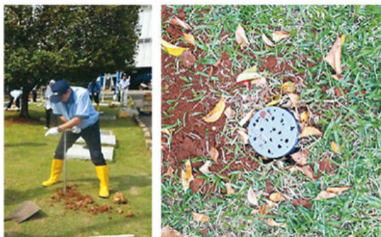
IEI employee digs hole for a biopore; a biopore in the ground
