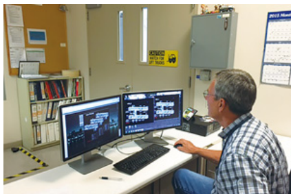
Checking the operations of the air conditioning system on a monitor
