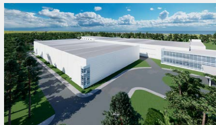
A new building for additional inkjet printhead production capacity is under construction at Epson Group company Tohoku Epson in anticipation of higher demand for printers, particularly commercial and industrial printers. The new building is scheduled for completion at the end of September 2025.
