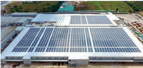
New factory in the Philippines with a rooftop mega-solar power plant with a maximum output of 3,000 kW of power (2017)
