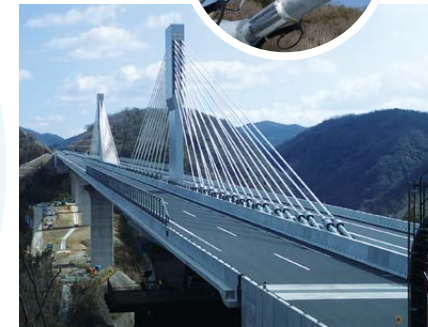
Shin-Meishin Expressway, Ikuno Bridge (NEXCO West Nippon)
