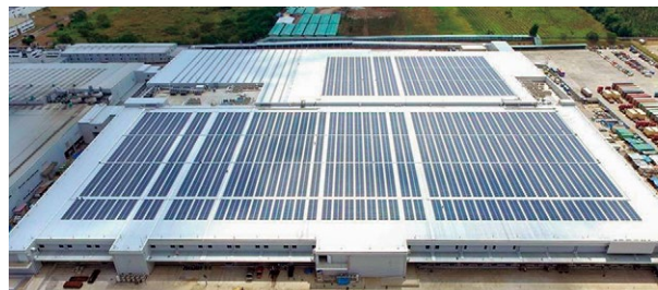
New factory in the Philippines with a rooftop mega-solar power plant with a maximum output of 3,000 kW of power (2017)
