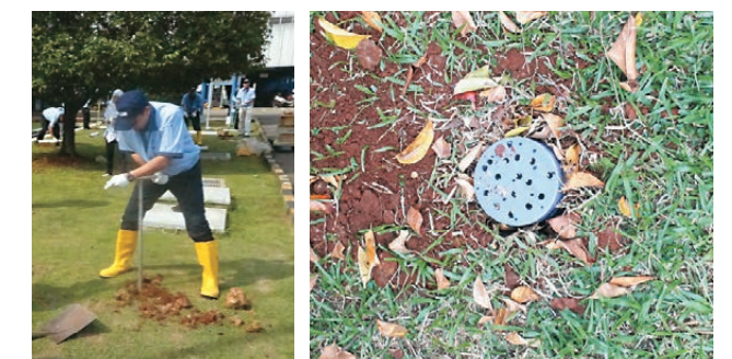
IEI employee digs hole for a biopore; a biopore in the ground
