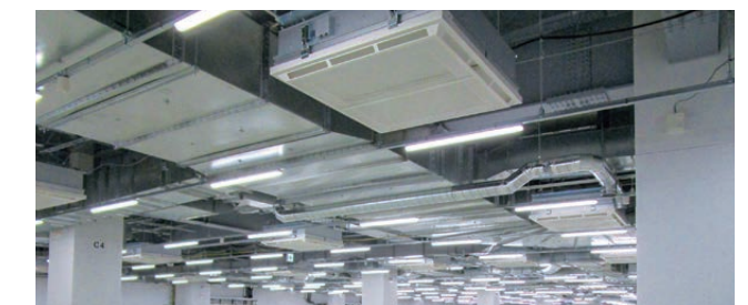
With no need for double ceilings or walls, air does not need to be circulated as often
