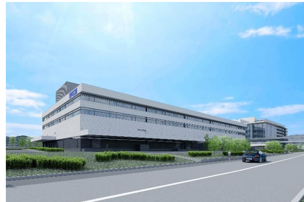
Innovation Center Building B in Hirooka (under construction)
