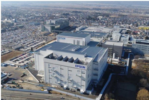
New plant (Building 9) at the Hirooka Office
