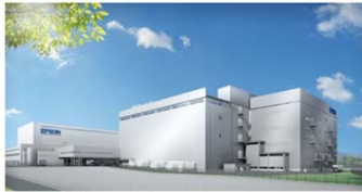
Inkjet printhead production & development functions to be strengthened in Hirooka (under construction)
